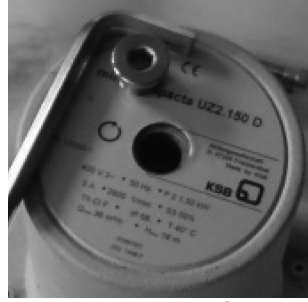
Fig. 16: Direction of rotation of the pump
